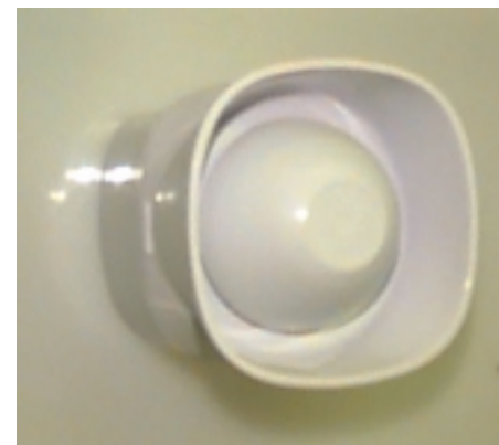
Figure 5: A typical egress beacon, a compact integrated sounding unit.
